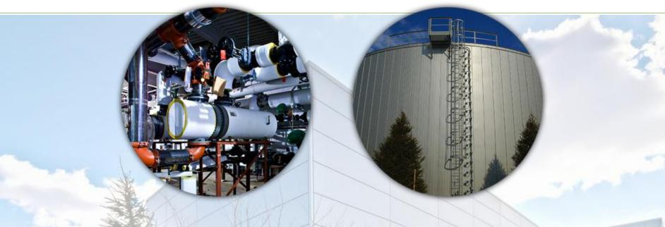
Recycling system provides electric and thermal energy from natural gas. Heat is created as a byproduct from the creation of electricity and is used to produce steam that heats the hospital.
