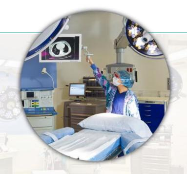
Instrumentation and equipment suspended from ceiling at eye level to improve visibility, mobility and safety and to reduce room turnaround time.
