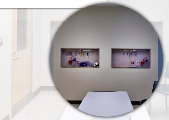
Control switches, gasses and supplies on the wall are covered by a polycarbonate panel to limit access to patients while allowing individual to see contents.
